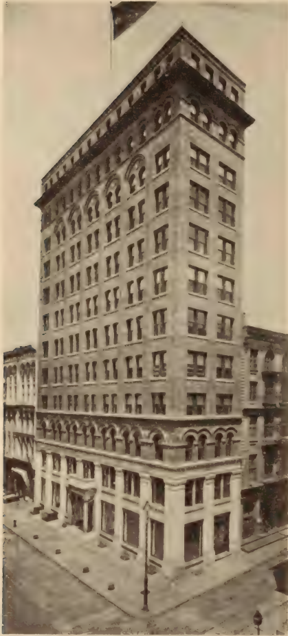
THE GRAHAM BUILDING.
